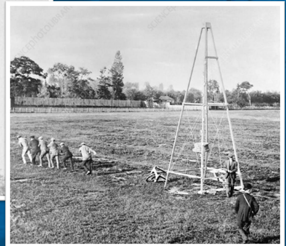
Top - The Wright Flyer 2. Right - The catapult launch system.
